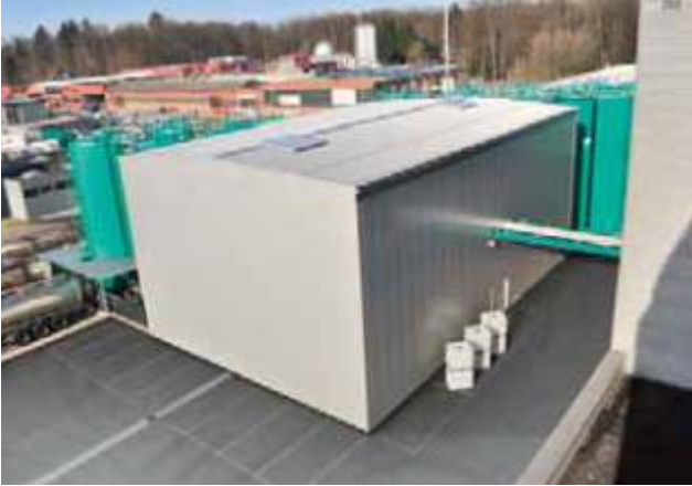
With the new fully enclosed storage tanks with pigging technology, Motorex emphasises once again its dedication to quality as leading Swiss lubrication technology specialist.
